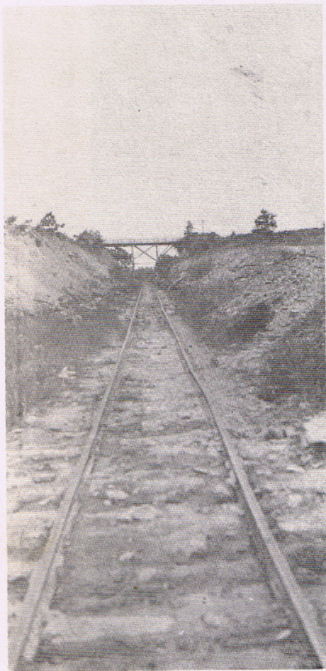
35 Foot Railroad cut at Sweeden leading to Black Gold Quarry. Highway 65 overhead bridge.
