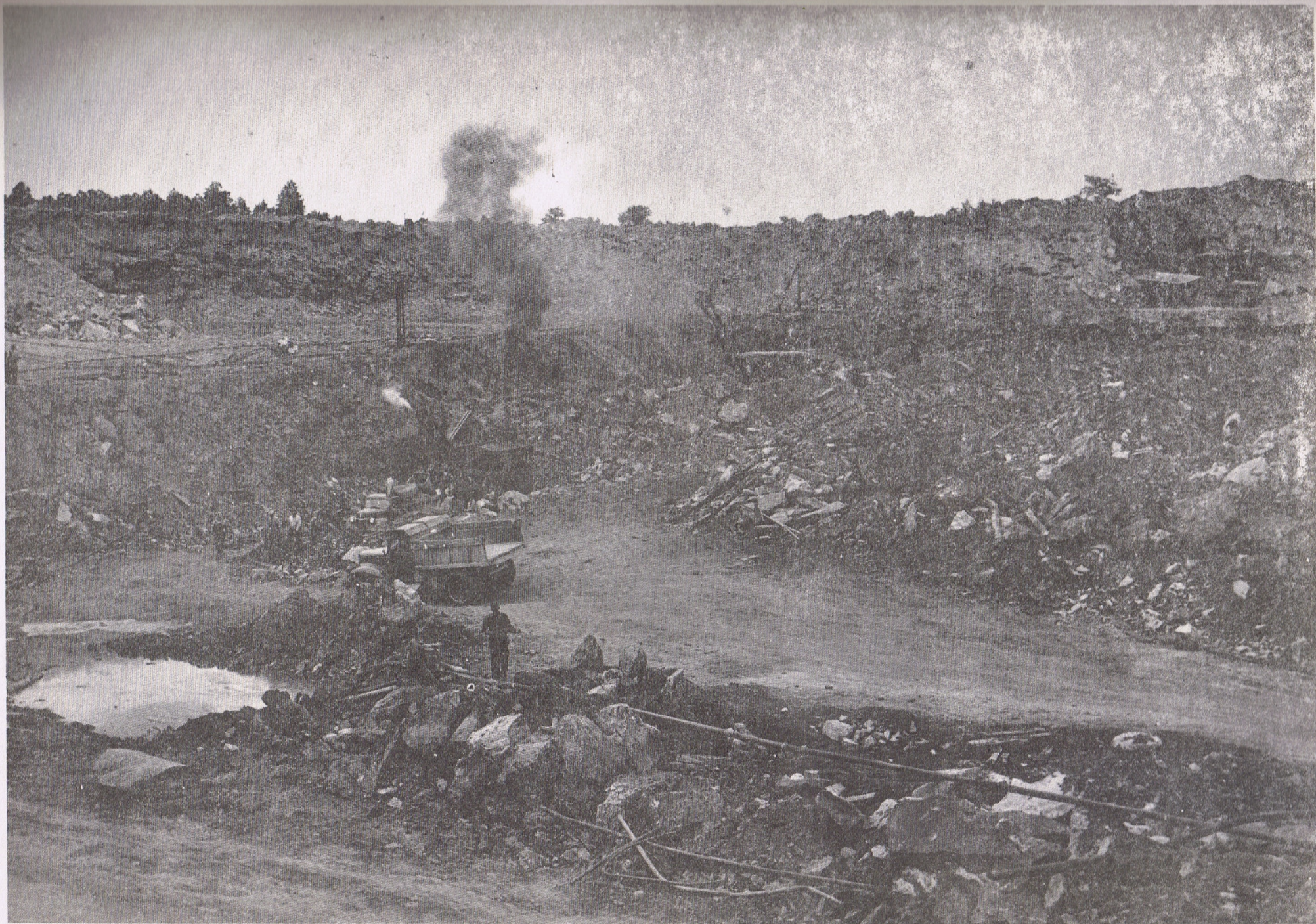
Asphalt Quarry at Black Gold.
